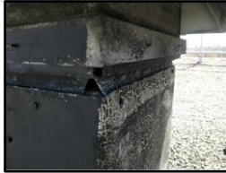
Improper Seating of Housing
