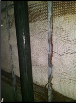
Missing insulation on cold water riser
