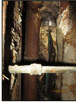
Damaged insulation on cold water riser
