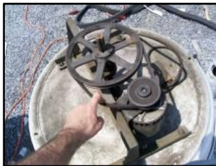
Loose or Broken Belts
