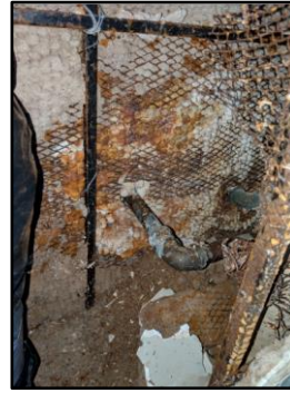
Missing insulation on cold water supply
